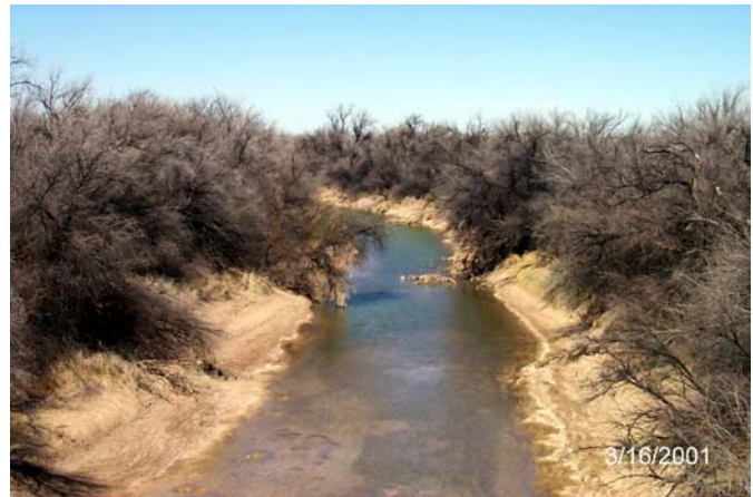
Mentone Bridge 18 Months Post-Treatment
